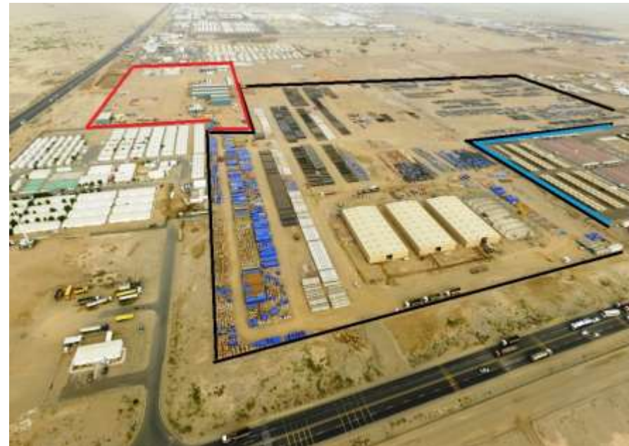
Laydown Area and Warehouse View
